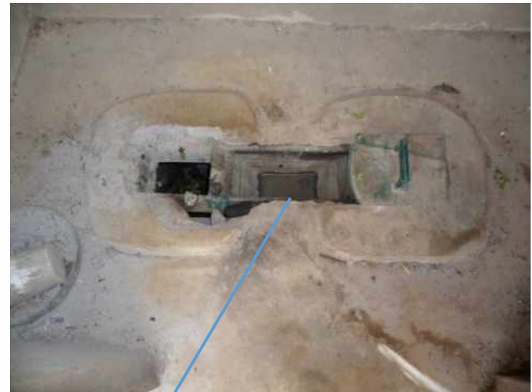
Blocked urine pipe
